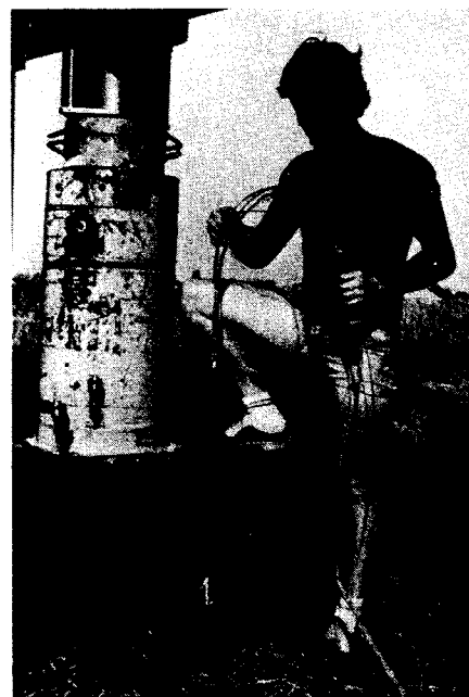
Figure 3. Removable extensometer being inserted into the sheet pile wall element of Merville.
