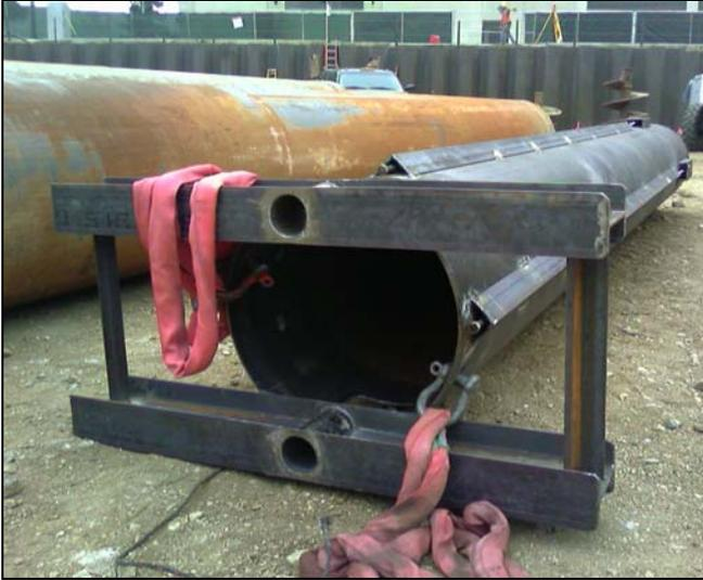
**Figure 6: Column installation template**
