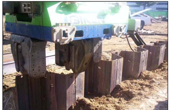
**Figure 2: Installation of sheet piles**
