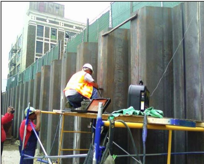
**Figure 9: Magnetic particle testing following welding of sheet pile**
