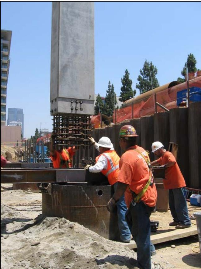
**Figure 7: Lowering precast gravity column into place**
